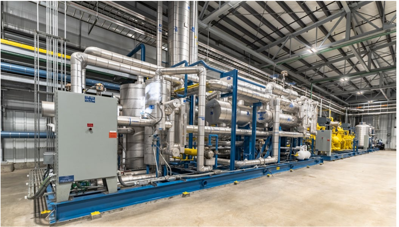
The liquefaction carbon dioxide skid for carbon capture/sequestration is at the Blue Flint Ethanol facility.
